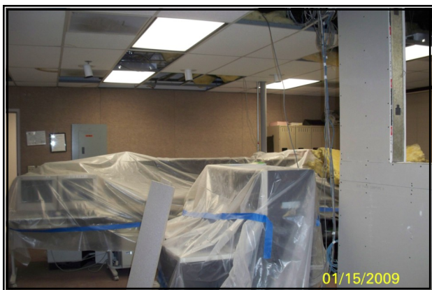
Alternate Site remodel in progress.
